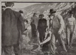
PUTTING IN THE STAKES.
